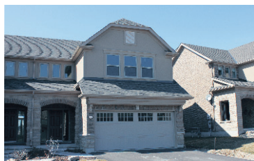
FINISHED TOP TO BOTTOM! $499,900
