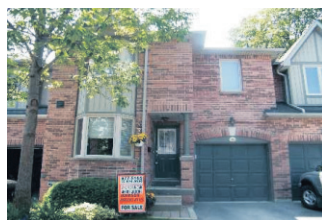
ALL THE WORK'S BEEN DONE! $389,000 Sandra Brianceau* 11-282-30 W2143865
