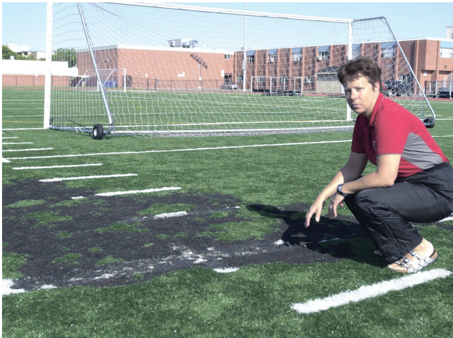
Georgetown Soccer Club president Alice Strachan surveys the damage at Kiwanis Field last week after several sections of the synthetic turf at the nine-month-old, $2.1-million facility were burned
