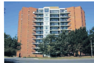
WELL MAINTAINED BUILDING-GREAT LOCATION $219,000 Ryan Green*
