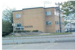
PROFESSIONAL SPACE - GREAT LOCATION $950/Month PresswoodTeam.com 11-135-30 W2078406
