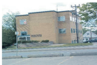
PROFESSIONAL SPACE - GREAT LOCATION $950/Month PresswoodTeam.com 11-135-30 W2078406
