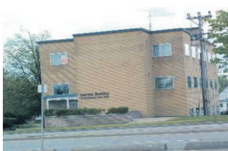
PRIME OFFICE SPACE $950/MONTH PresswoodTeam.com
