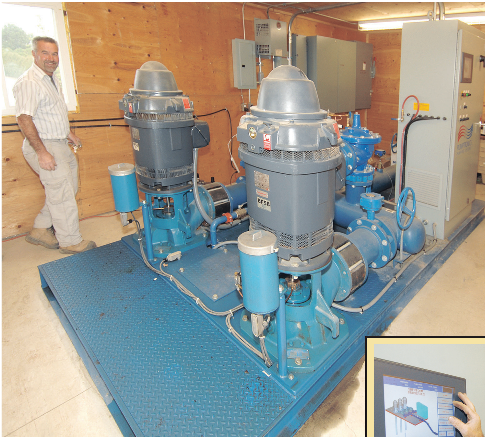
Left: Sheridan's irrigation supervisor Steve Deschenes checks out the nerve centre of the irrigation system, which consists of two 60-horsepower pumps that can each move 1,100 gallons of water a minute, through a 14-inch main pipe in a computer-monitored pump house, which then irrigates more than 600 acres of Sheridan's farmland.
