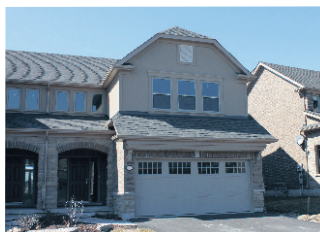
FINISHED TOP TO BOTTOM! $499,900
