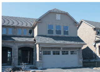
FINISHED TOP TO BOTTOM! $499,900
