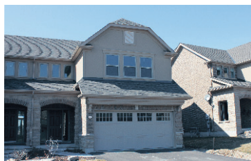
FINISHED TOP TO BOTTOM! $499,900
