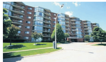
SUPERB WELL MAINTAINED PENTHOUSE $227,500
