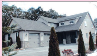
PIECE OF PARADISE BACKING ONTO THE 12TH GREEN WITH CUSTOM BUILT 3600 SQ FT. RESIDENCE $999,000
