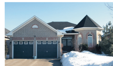
54 Johnson Crescent, Georgetown Sunday, March 6, 2:00-4:00 $509,950
