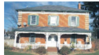
COMPLETELY RENOVATED CENTURY HOME
