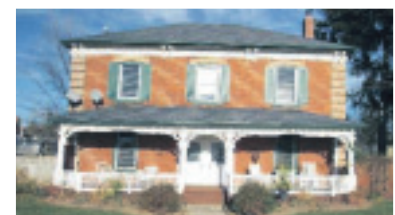
COMPLETELY RENOVATED CENTURY HOME
