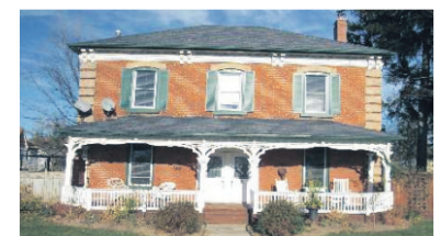
COMPLETELY RENOVATED CENTURY HOME
