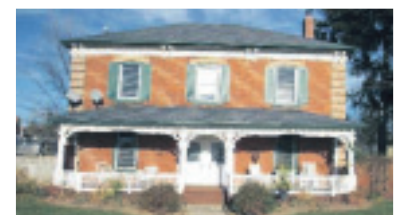
COMPLETELY RENOVATED CENTURY HOME
