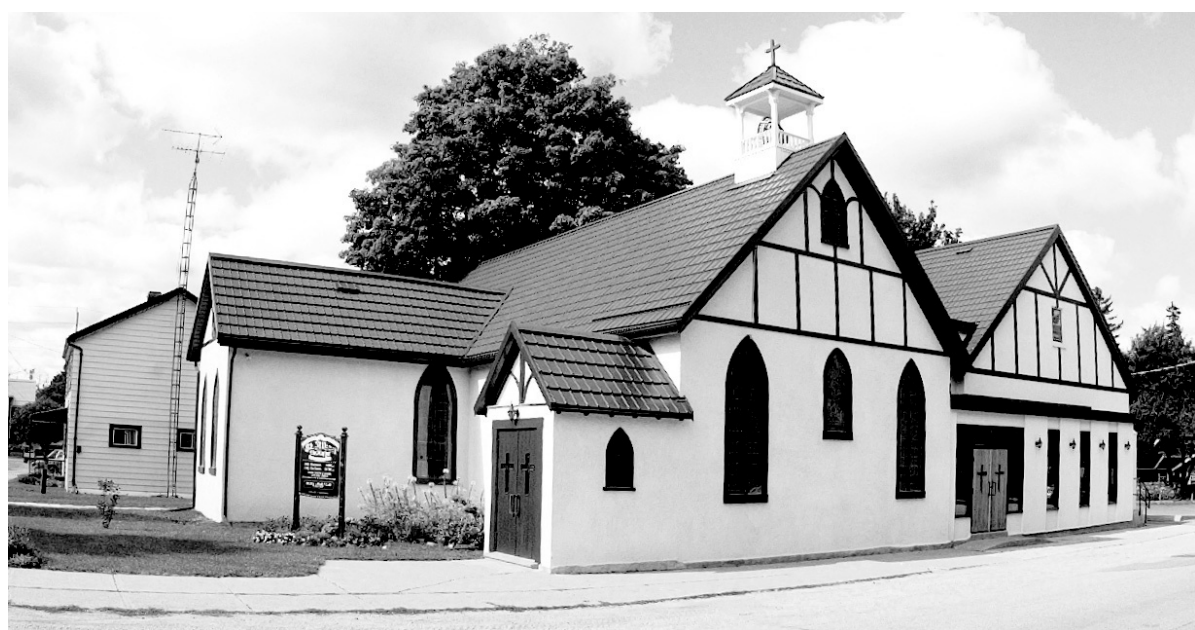
Above: St. Alban's Church, located at 19 St. Alban's Dr. in Acton, was built in 1872 and the Parish Hall was built in 1959. The Luxton Memorial Hall, which was built almost entirely by volunteers, was named after the rector who was in residence around 1950. File photo
