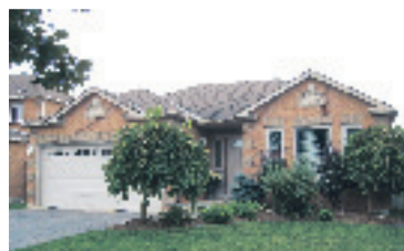
BIGGER THAN IT LOOKS-4 LEVEL BACKSPLIT $429,000
