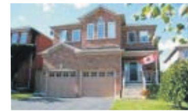
SUPERB STREET IN GEORGETOWN SOUTH $579,900
