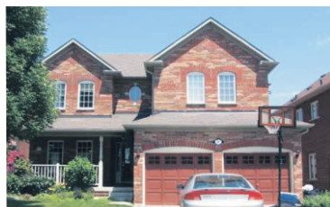
STEWARTS MILL LOCATION $519,900
