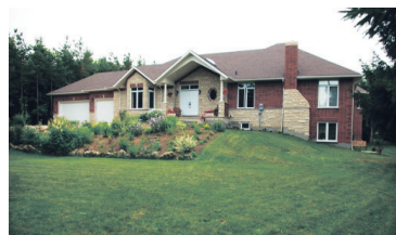
QUALITY WORKMANSHIP ON 1 AC $775,000
