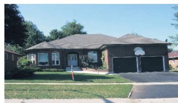
BUNGALOW WITH W/O BASEMENT
