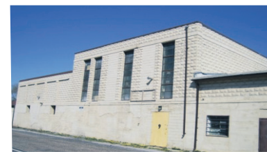
INDUSTRIAL UNIT IN HEART OF GEORGETOWN David Burland* 10-168-30 W1844823
