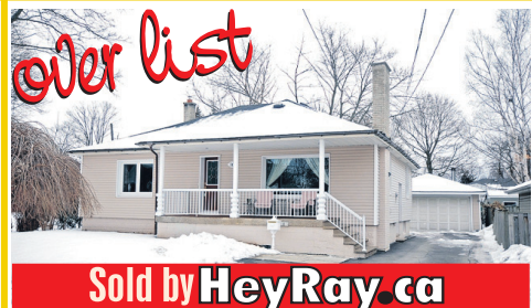
over list Sold by HeyRay.ca Blended Family? Perfect layout for blended, extended or family with teenagers! Updated & renovated 3+3, 2 bath bungalow on gorgeous lot with detached garage - walk to GO Station & downtown. $359,900.00 MLS# W1799644
