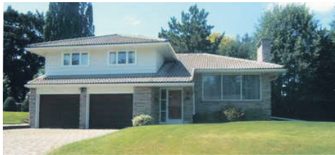
CUSTOM BUILT HOME IN PARK AREA $569,000 09-364-30 W1679220 Iris Irwin*
