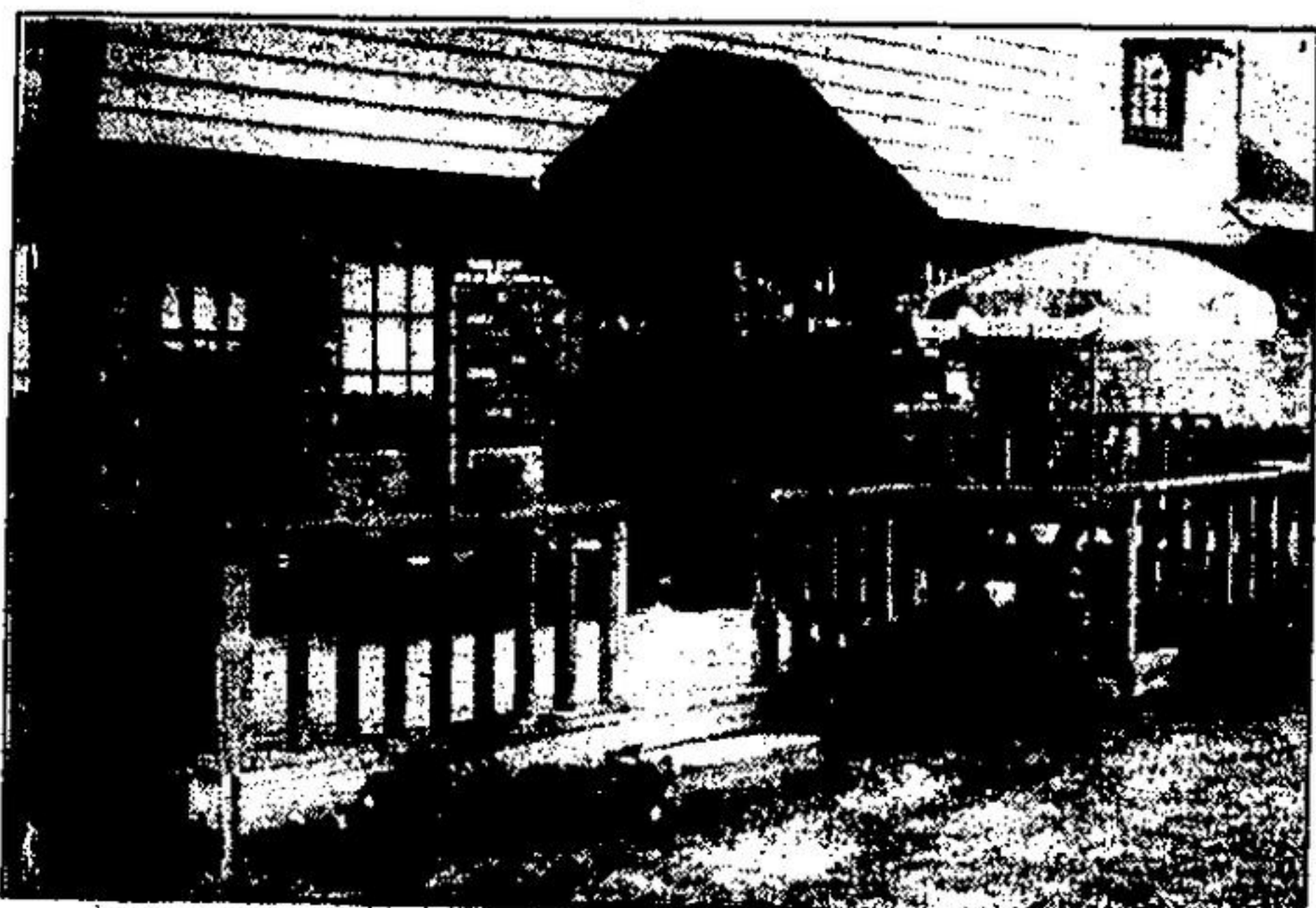
DECKS, RAILINGS and other exterior structures built with pressure-treated wood need waterproofing to prevent moisture damage like warping, splitting and cracking. Protect your investment with the proper care and you can maintain its beauty and durability for years to come.
