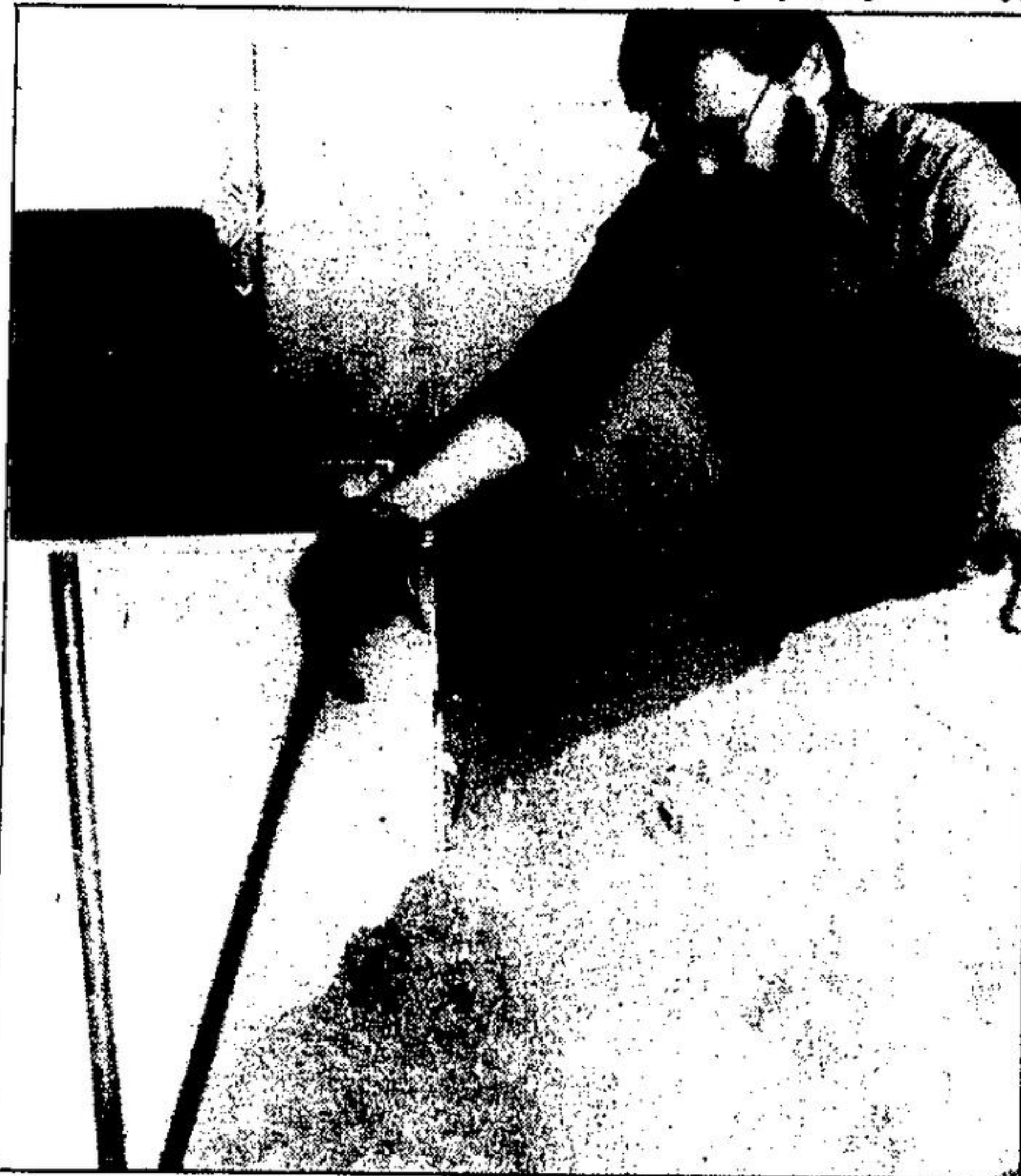
Halton-Peel MP Garth Turner has been busy recently renovating his constituency office in Georgetown. Mr. Turner, along with his wife Dorothy and some volunteers, are replacing the floor and knocking out some of the walls. Mr. Turner wants more space so he can hold committee meetings in the office. This will save taxpayers money because currently a space has to be rented out everytime a meeting is scheduled, Mr. Turner says. (Herald photo)
