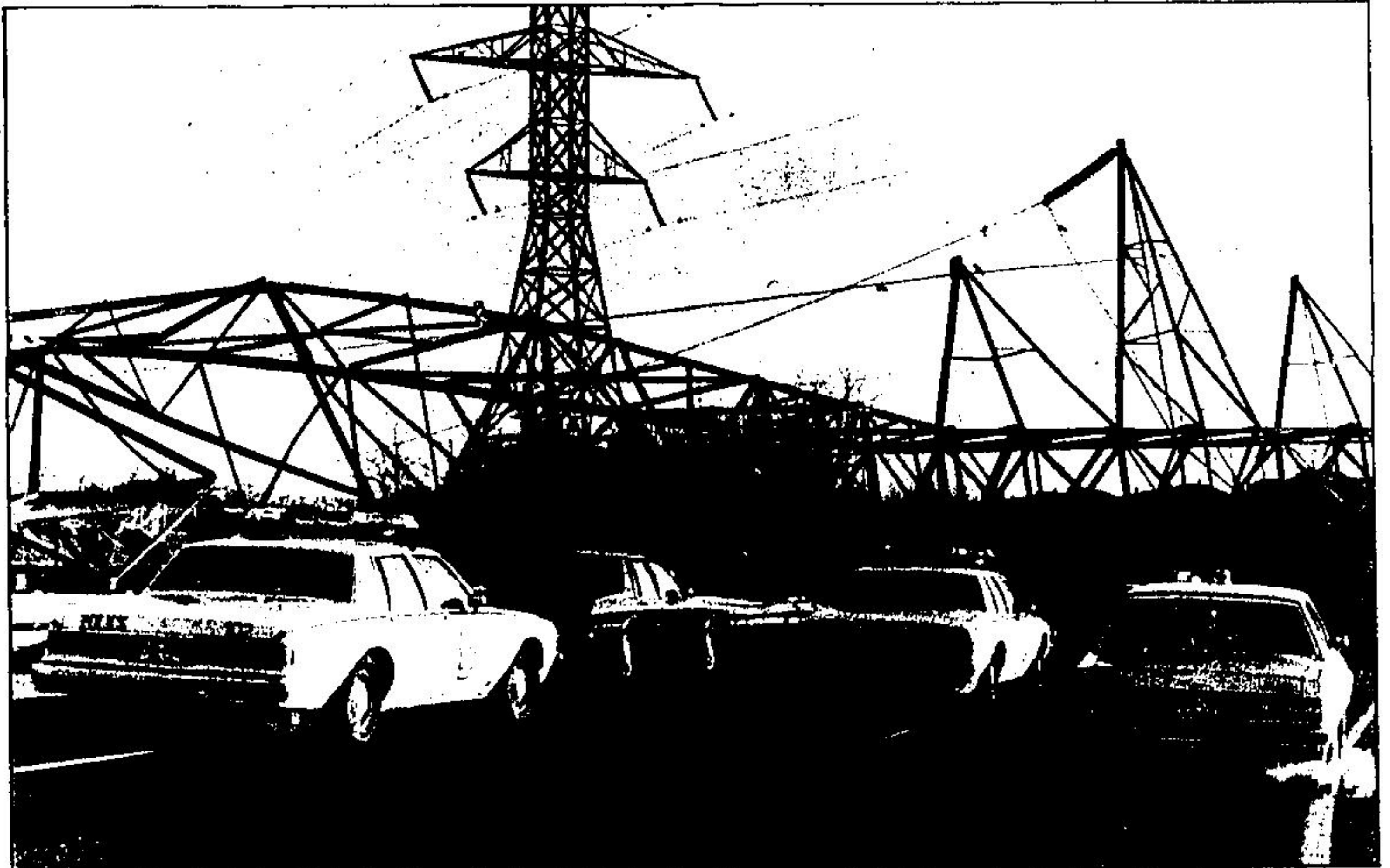
Power was off for over eight hours after a hydro transmission tower came crashing across an off-ramp along Hwy. 403. Officials suspect vandalism as the cause for the incident which led to traffic problems and loss
