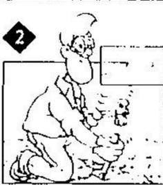
Wearing goggles to protect your eyes from flying fragments, break up large areas of spalled concrete surface with a small sledge hammer, let the hammer drop of its own weight rather than swinging it hard against the surface. For small areas use a ball peen hammer and cold chisel. Sweep up dust and debris using a stiff wire brush, if necessary, to dislodge any small fragments.
