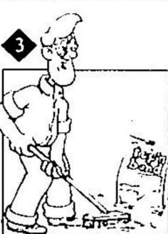
Chip away all cracks to about 1/2 inch below the surface using a cold chisel and ball peen hammer. Flare the walls out slightly making the bottom wider than the opening at the top. Wear goggles and gloves while doing this to protect yourself from flying fragments. Fill these cracks with Sakrete® Sand Mix available from your local building supplies retailer. Allow these repairs to cure for 72 hours before you begin resurfacing.
