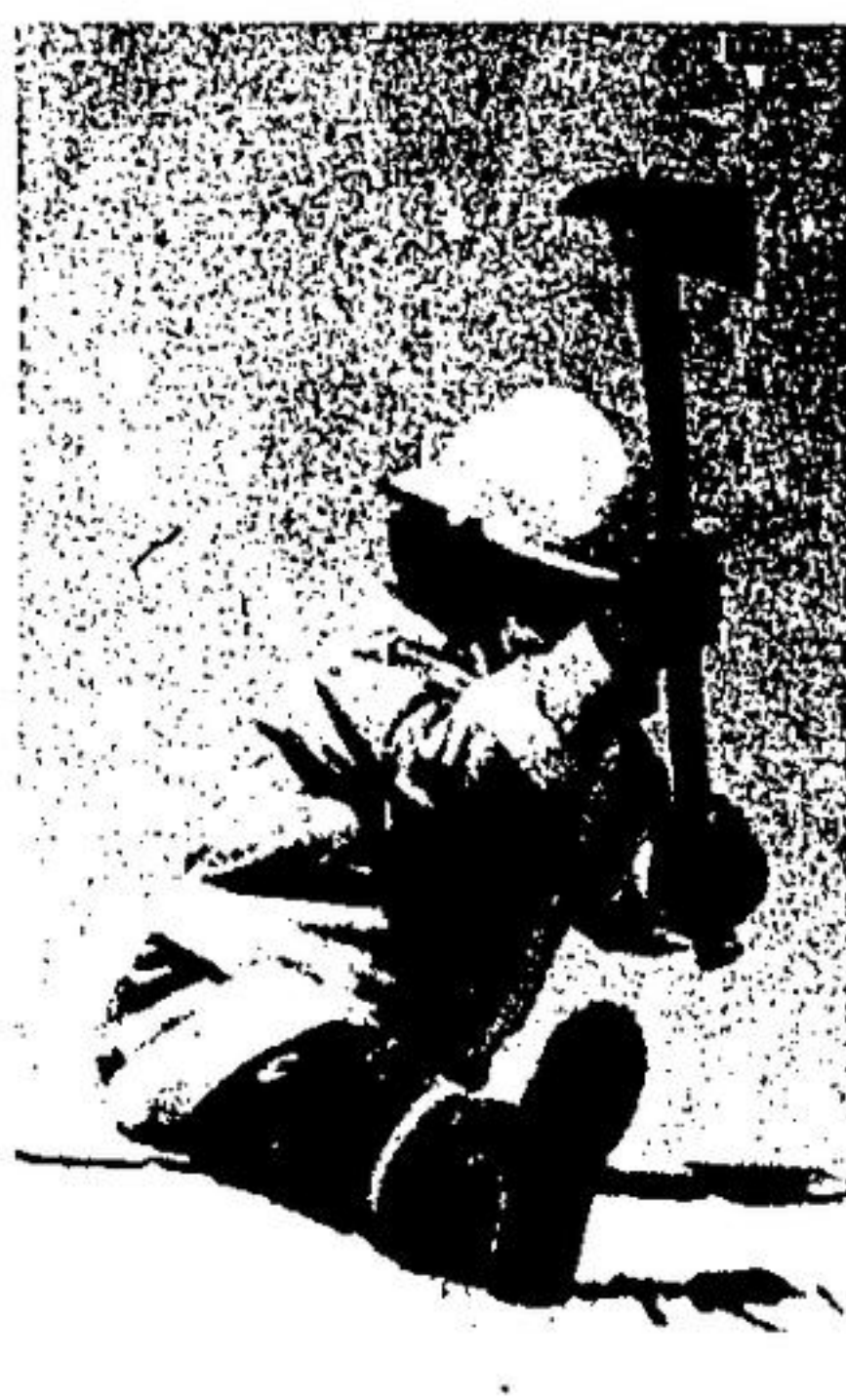
For a change the Georgetown fire department got to start a fire on March 6. Here, they prepare an old building to set a blaze before putting the flames out. But one fireman drew the assignment of balancing himself on top of the building to knock a hole through the roof. (Herald photo)
