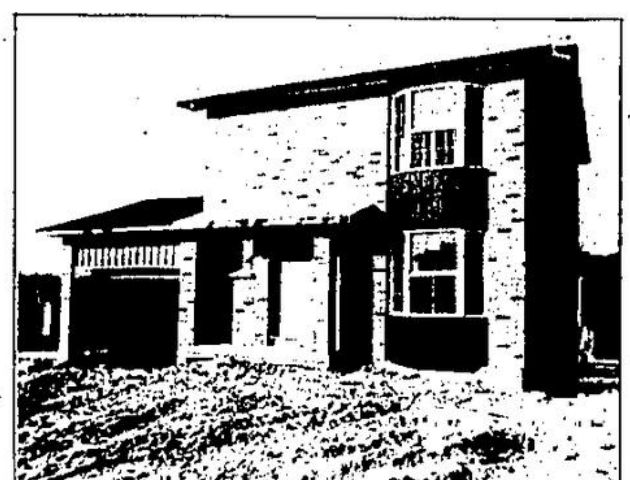
BRAND NEW, $99,900 — Lovely 2 storey, 3 bedroom home in quiet court, 1 1/2 bathrooms, bay windows, extra large master bedroom and walkout are only some of the features. For a personal inspection call Mal Dodge, 877-5213. 6196
