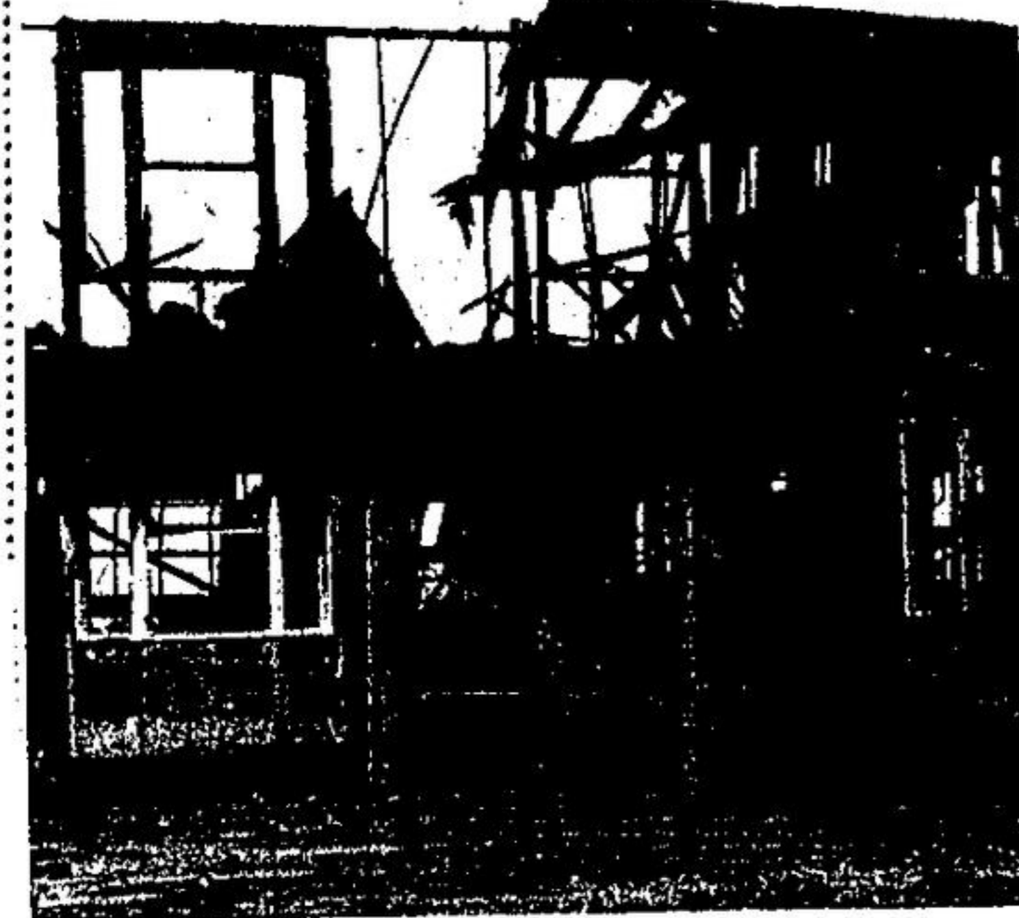
All that remains of this house is the charred frame. Four unfurnished homes located behind the Georgetown Plaza were burned in a blaze that began at 4:48 a.m. last Wednesday. The Halton Hills Fire Department is listing the blaze as a suspicious fire. (Herald photo)
