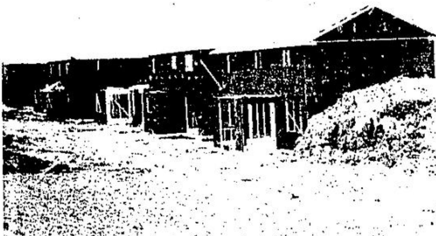
Construction is well underway at a new subdivision behind the Georgetown Market Plaza. Roofs are now in the process of being erected on several of the units.
