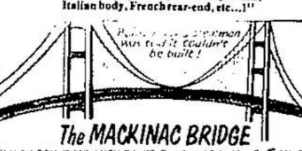
WHICH CONNECTS MICHIGANIS 2 PENINSULAS, IS S MILES LONG, COUNTING THE APPROACHES! AROUND 10,000 MEN WERE INVOLVED IN THE CONSTRUCTION OF IT, THE BRIDGE CONTAINS 4.8 MILLION RIVETS AND ABOUT A MILLION BOLTS. 85,000 BLUEPRINTS WERE DRAWN. EVERY TOLEPANCE WAS MET WITHIN 1/32 OF AN INCH. OVER A MILLION TONS OF STEEL AND CONCRETE WERE USED, 9/10 OF WHICH ARE UNDER WATER.
