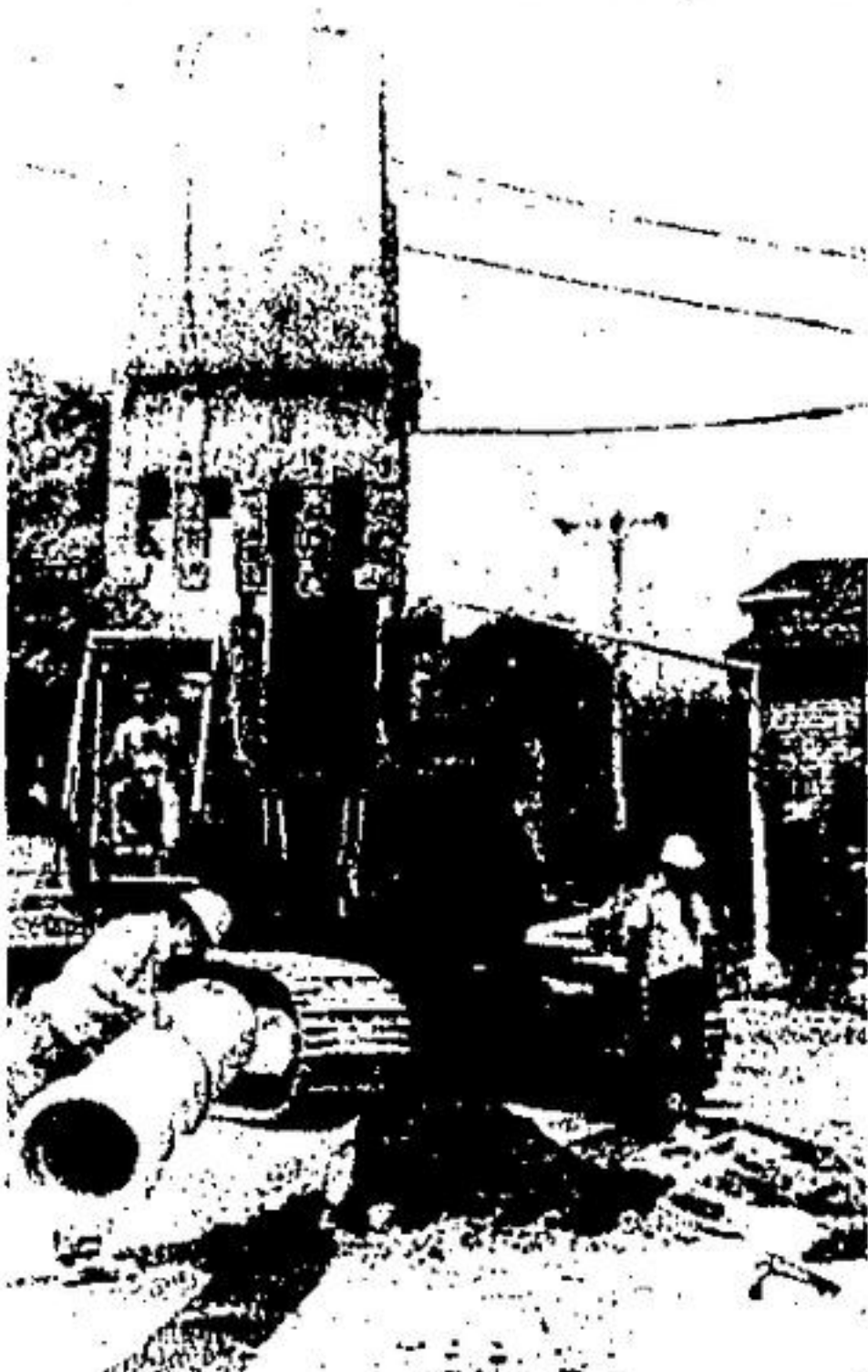
Mill Street, Georgetown is reconstructed between Main and Mill Streets as part of a downtown improvement project.
