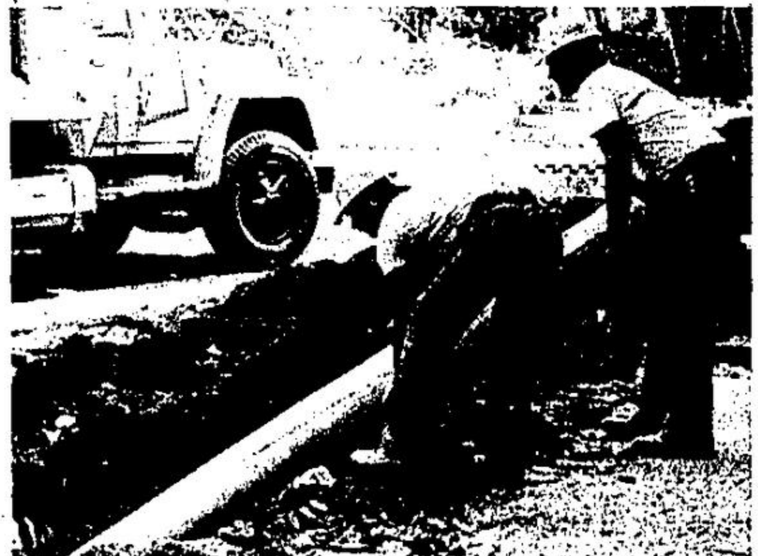
Sweat pouring off their brows, construction crews settled storm, sanitary and water mains under Murdoch, Albert, McNabb and Queen Streets, last week. Temperatures soared giving Georgetown the summer heat it missed last year. (Herald photo)
