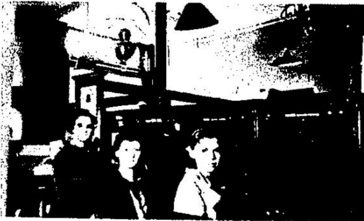
Staffing the switchboard in Halton Hills: two enterprising Acton inventors deserve the honor for first bringing the telephone to north Halton.
