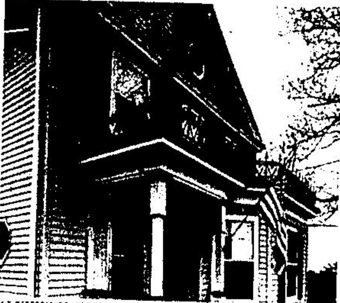
ALUMINUM SIDING AND TRIM were used to preserve the authenticity of this old Victorian gem. The surface was covered with double-four-inch aluminum panels which match the original clapboard, and aluminum coil stock was formed to follow the contours of trim such as the octagonal window casings, porch scalloping, ceiling and fascia. Old grillwork on second story was repaired and painted.
