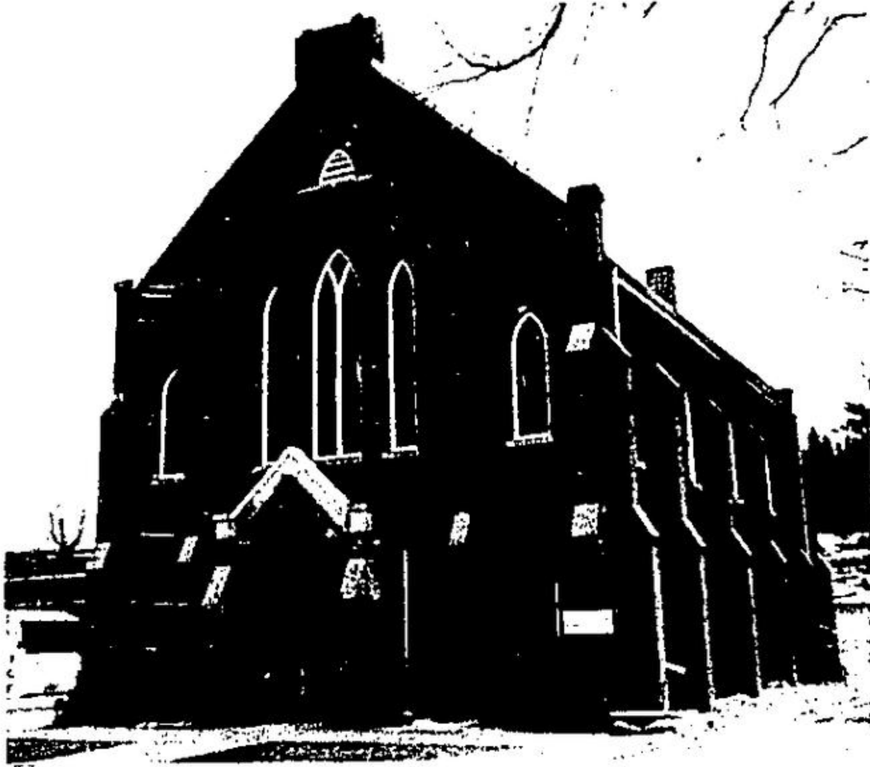
The long narrow windows facing onto Norval's stretch of Highway 7 give away the age of this church. The Norval United Church was built in 1889, a fact that's recorded in the stained glass windows. Rev. Walter Ridley, minister at the church since 1968, also cares for the Huttonville parish in Brampton and the Home Church parish in Caledon. A theology student helps Rev. Ridley in his work. (Herald photo)
