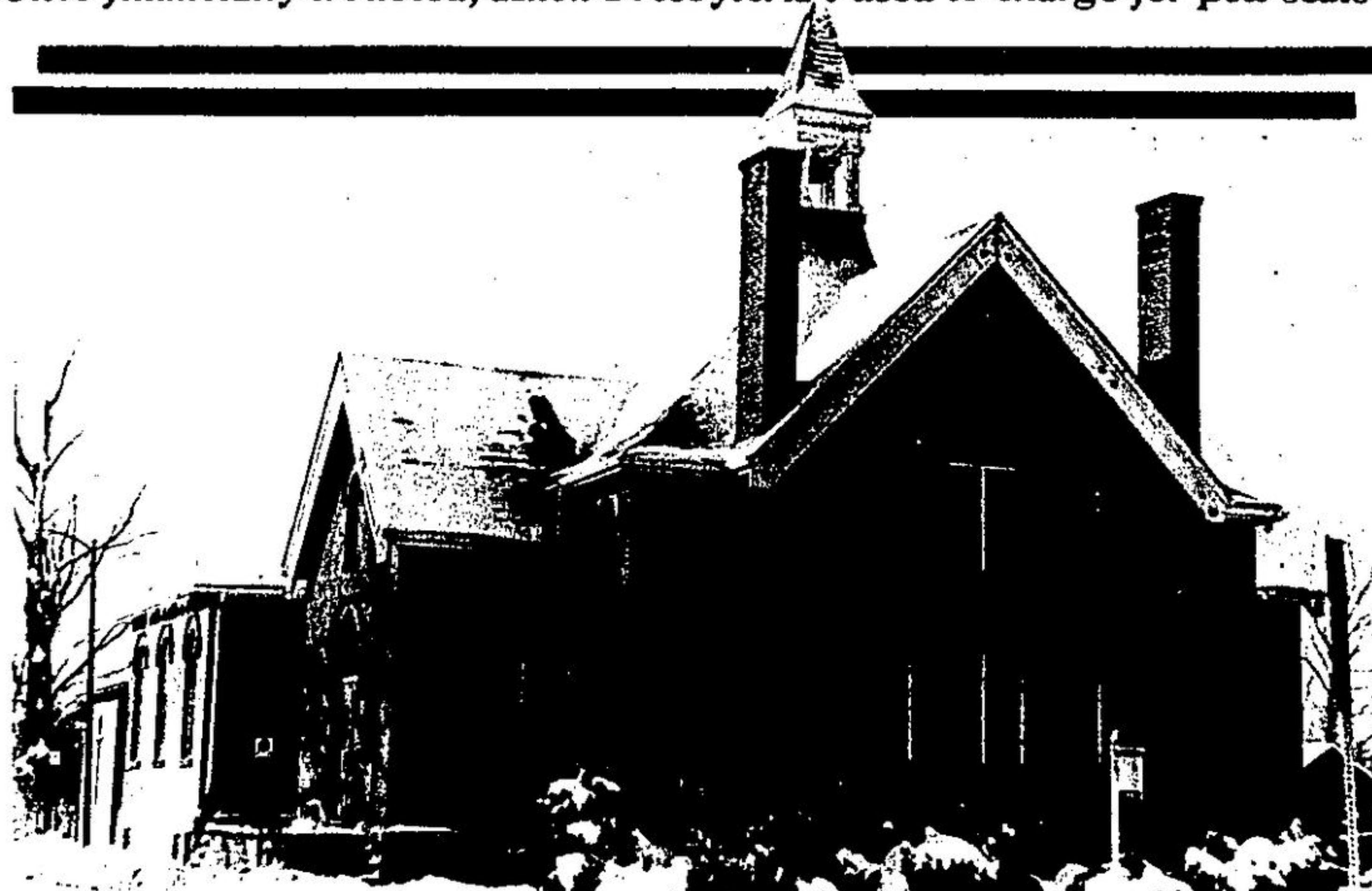
Built in 1884, the Knox Presbyterian Church building on Acton's Main Street at Knox Avenue is the second church building for the congregation that organized itself in 1845. Veneered with pressed brick, the building rests upon a stone foundation. Semi-circular arches, front and side gables, an ornamental turret and slated roofs distinguish the almost 90 year old building. The very
