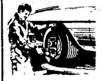
Here's what we do Adjust camber, caster and toe-in to manufacturer's specifications . Adjust torsion bars . Inspect front end suspension. springs, shocks and aleering assembly
