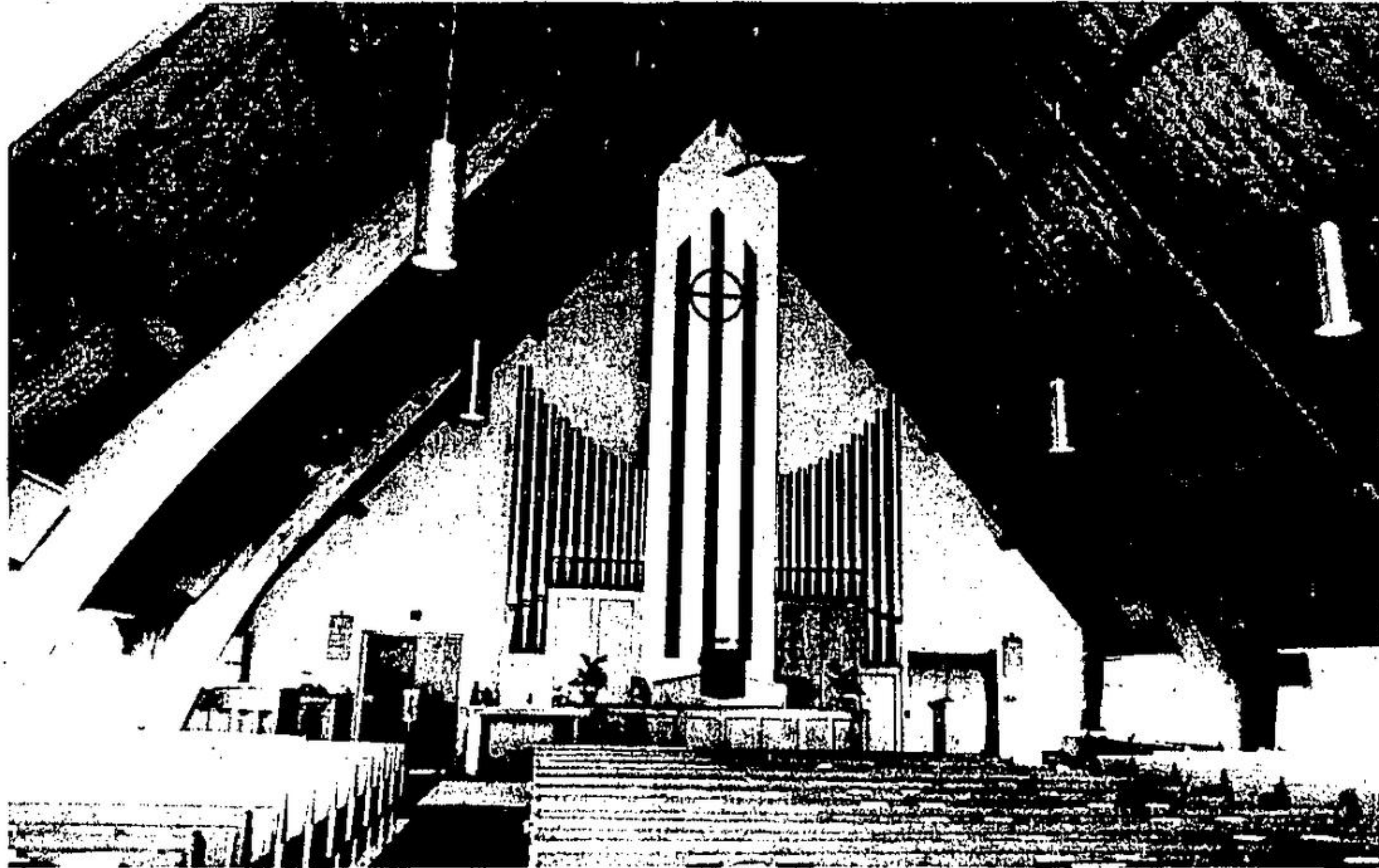
Broad wooden arches meet at the centre of a high roof in the Christian Reformed Church in Georgetown. Reverend John DeJong said buildings aren't built this way anymore because although it's architecturally attractive, it isn't economically wise. The high ceiling means all the hot air rises above where it can be useful. Fans have been installed to circulate the warm air. (Herald photo)
