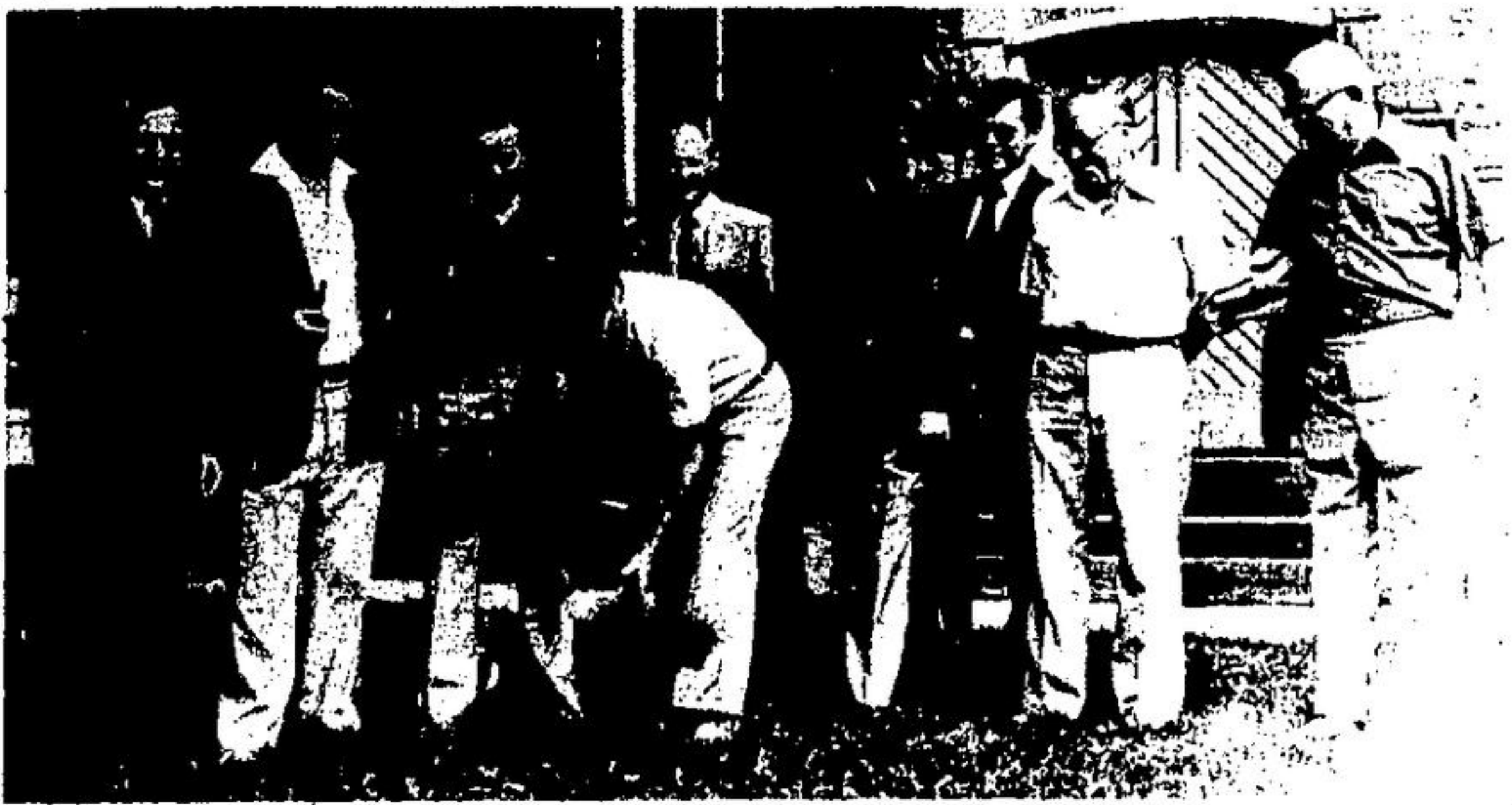
Mayor Pete Pomeroy is joined by members of the library-cultural centre building committee as he cuts the first turf to launch construction of the $1.3 million facility last Tuesday. Much of the town's share of the building cost has already been raised from GLT seat plaque sales and organizers aren't too worried about paying for the centre thanks to the success and popularity of the campaign. Pictured here from left are Derek Woynes, Coun. Roy Booth, Ab Tennant, Dick Howitt, Keith Wagland (architect), Rex Heslop Jr., Coun. Ross Knechtel and Coun. Pat Patterson.
