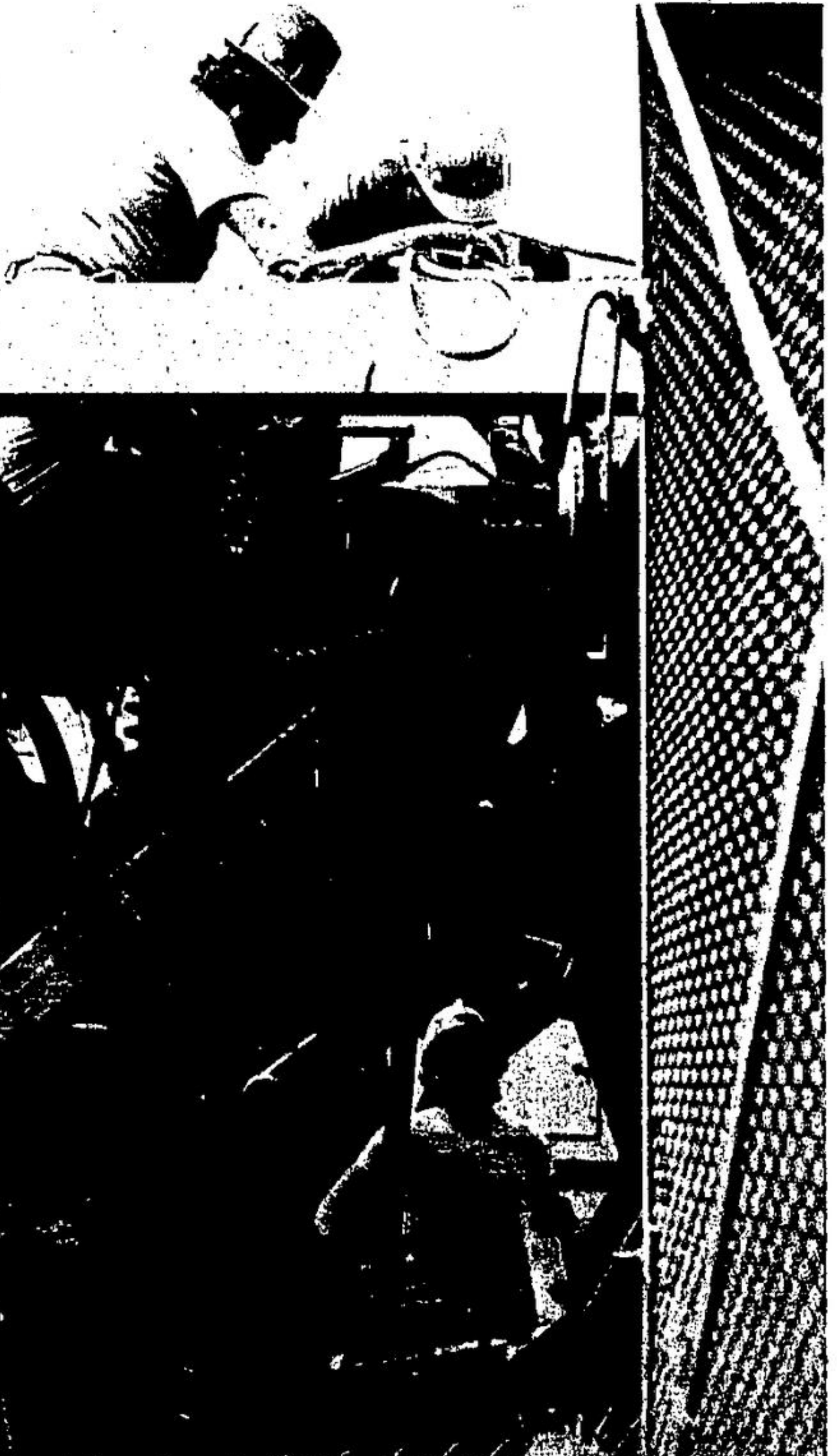
Not all the work on the site is directly related to the stringing of the lines. The machines must be maintained in good working order, and two of the men are shown here working on one of the tensioners, which sets the tension of the lines.
