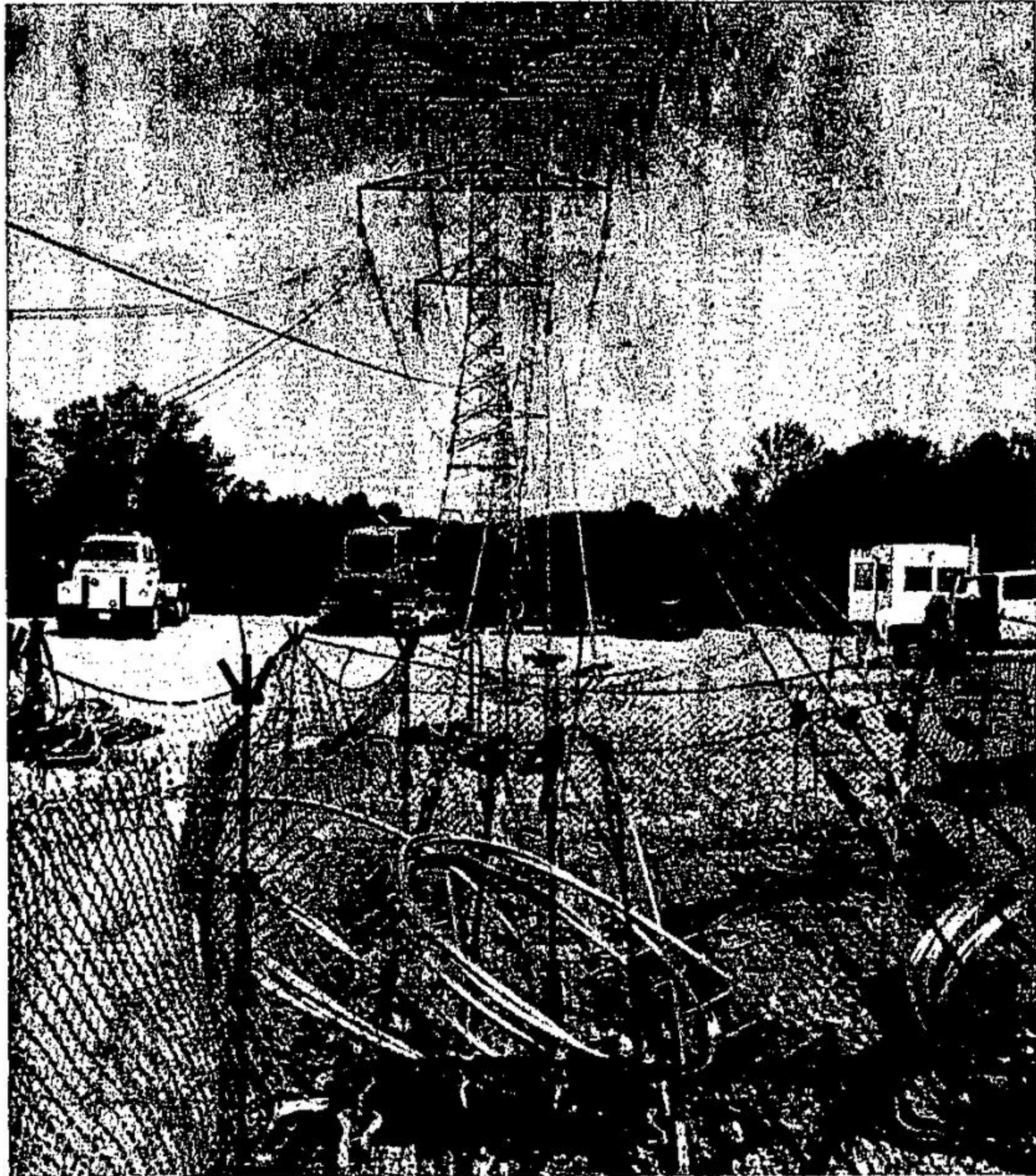
The conductor ends drop from the arms of the tower to the ground where they are secured in grips. Once the next section of line is in place, the ends will be spliced together with splicers,
