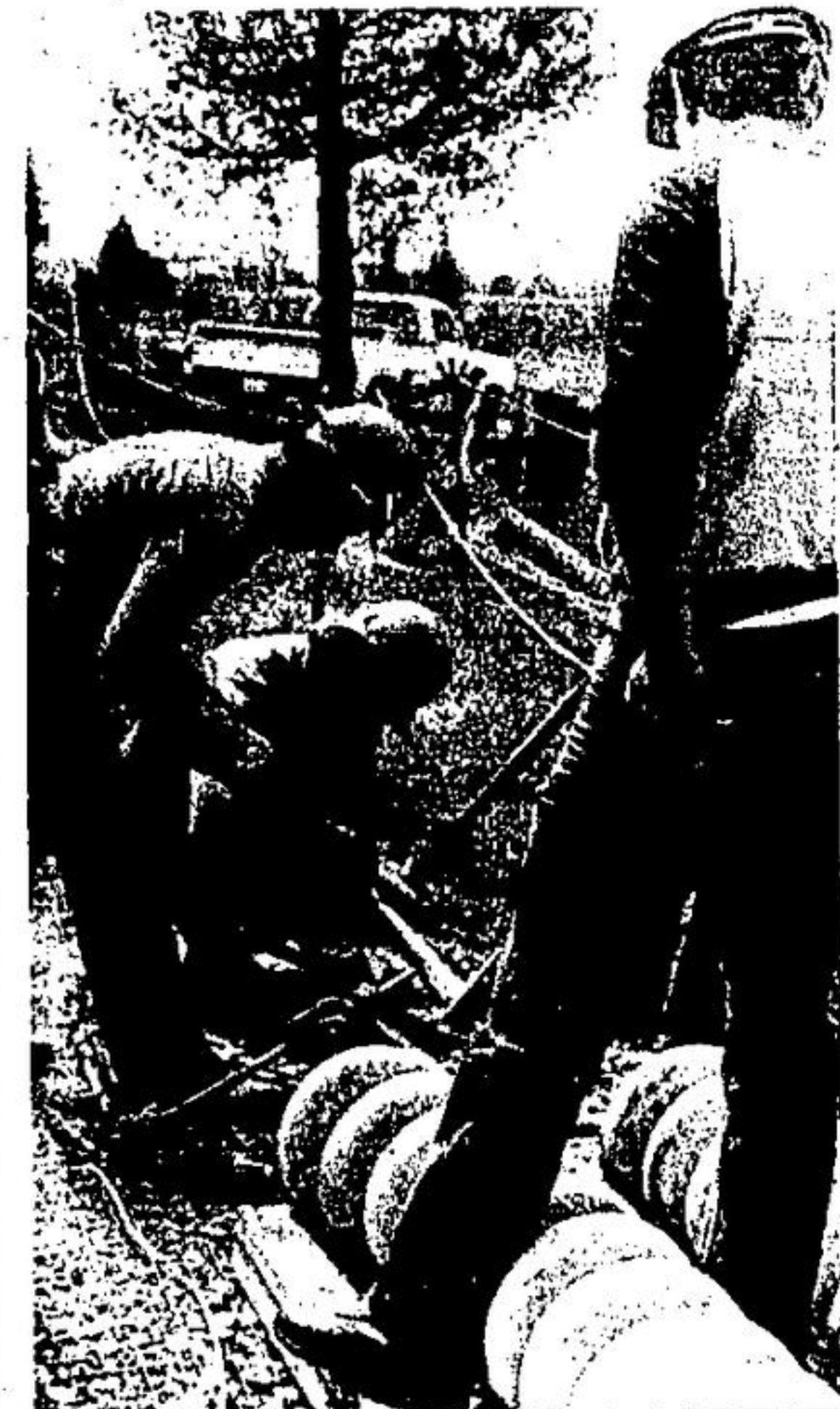
Lines construction workers connect the insulators to the conductors. The insulator is then attached to the tower, after being hauled up by a pulley and moved into position by a bulldozer.
