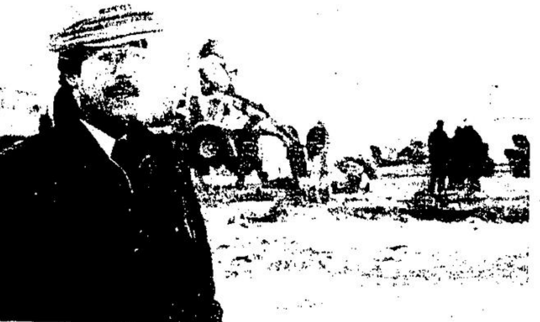
Ontario Hydro community relations officer Chris Taylor stands before machinery being used by the utility to erect the remaining 50 towers in Hydro's 100-mile long super-corridor. Mr. Taylor spent much of the past week attempting to soothe anxious landowners and angry corridor opponents while at the same time defending Hydro's right to expropriate easements. (Herald photo)
