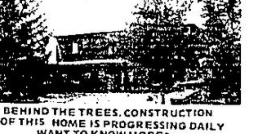
BEHIND THE TREES, CONSTRUCTION OF THIS HOME IS PROGRESSING DAILY WANT TO KNOW MORE? CALL ALICE POKLUDA
