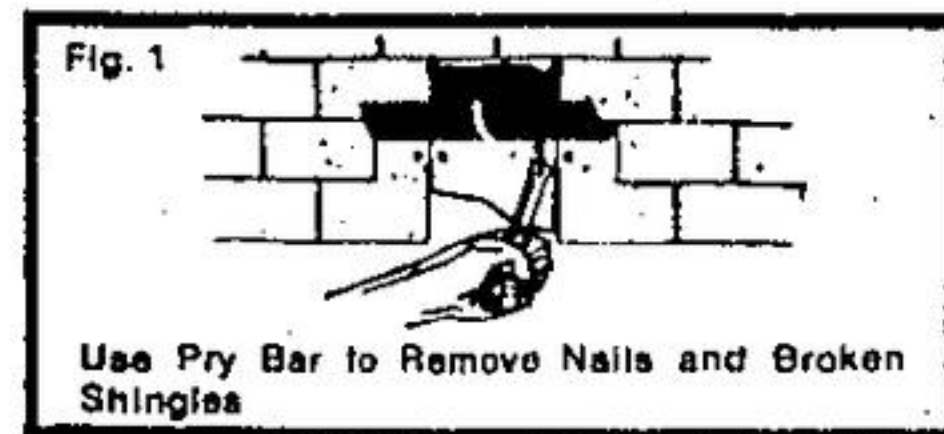
Use Pry Bar to Remove Nails and Broken Shingles
