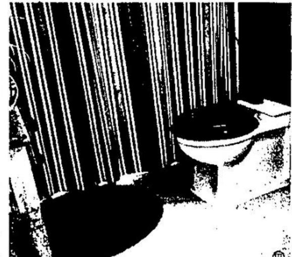
NUMBER ONE WATER SAVER—The two-quart Mi croppor LF-210 toilet is shown here installed in a typical residence. The unit has no water tank as such, and operates at a low noise level. This installation features a custom toilet seat that matches the color of the shower curtain. Made of vitreous china, the unit is streamlined and modern. It can be installed easily without complicated or costly plumbing modifications.
